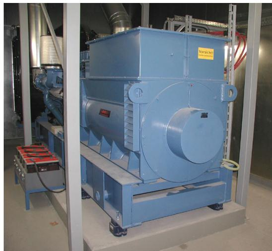
III.9: Vibration-isolated set-up of a power unit,
